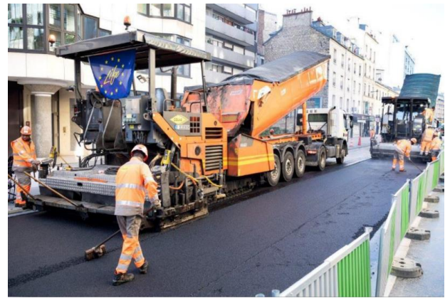
Figure 5 Frémicourt street with new asphalt mixes, October 2018.
